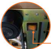
The Main Switch is located on the lower right part of the machine, near the front foot.
